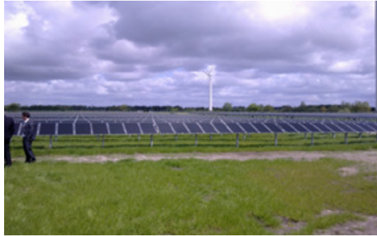
No.1 View from the front
